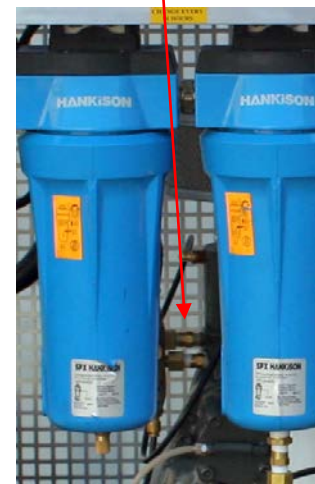
On/Off Flow Valve Handle in Off Position
