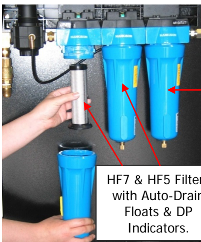
HF1 Filter with Manual Drain – Should not Contain Moisture
