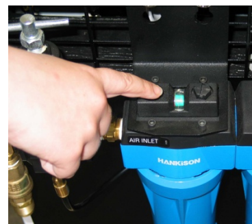
DP Indicator Changes from Green to Red as Filter Ages. Do Not Use When Red.
