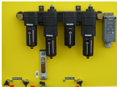
Manual Condensate Drain Valves
